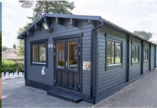
Finished Building after application of stain sealant
